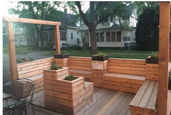
Build a small outdoor patio or park for neighborly gathering
